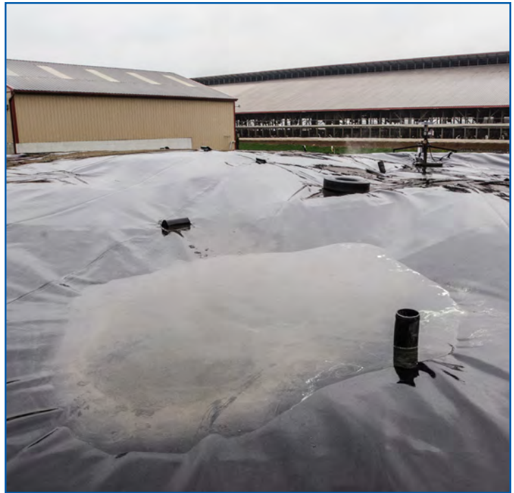
Rainwater and other debris collect in puddles on the cover of a manure lagoon located at a Pennsylvania dairy.
