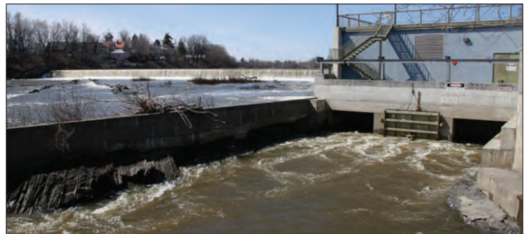
Algonquin's St. Hyacinthe Power Generating Station in Québec, Canada.
